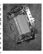
Install the stone to the sub-wall using acceptable industry practices. Remove the box setting fixture. Reattach the front section to the back section of the metallic box. The metallic outlet box assembly is now ready for the trim components to be installed.
