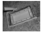
Re-insert the outlet box assembly, pushing down firmly until the adhesive pushes through the perforations in the mounting ring flange. Once the outlet is seated in the opening put a weighted object on the front collar, and allow the adhesive to cure. The stone panel assembly is now ready to be attached to the wall and the two portions of the metallic outlet box secured together.
