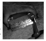
Remove the outlet box assembly from the stone. Then, using a strong adhesive such as Liquid Nails for Stone & Masonry, Superior Poli-Epoxy paste or 3M Scotch-Weld DP100 epoxy, lay a bead around the opening in the stone.
