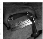
Pre-drill pilot holes through the perforated mounting ring and attach using #6 (or larger) wood screws of appropriate length. Attach the front box section to the wood paneling.
