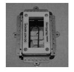
Important: National Electric Code (NEC) Section 314-23 requires that an electrical enclosure be rigidly mounted to the structure by mechanical means. The cutout above is optimized to insure a mechanical coupling of the electrical box perforated collar between the primary wall surface and
