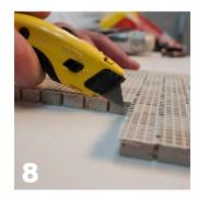
Cut tile - grinder or tile saw may be needed to cut individual tiles.
