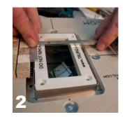
Lay in tile dam with plastic fixture and determine amount of shims needed. Tile dam is best fitted slightly lower than the tile height. Remember to compensate for mud behind tile.
