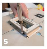
Fasten the tile dam using the four mud dam screws. Be sure to use a low torque setting so that the tile dam is not distorted. Also, if longer screws are needed, any standard #6 pan head screw can be used.
