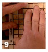
Set tile - being mindful of keeping an equal grout line around device.
