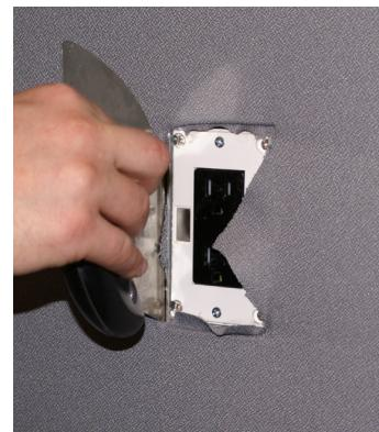
Next, use a putty knife, or similar, to tuck the fabric between the outside of the enclosure box and the MDF.
