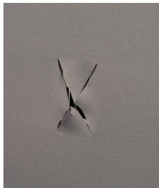
Using sharp scissors, cut an "X" from the corners of the TRUFIG opening.
