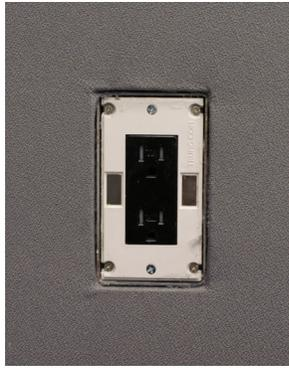
Once finished tucking the fabric, the fabric around the opening should be even and tight.
