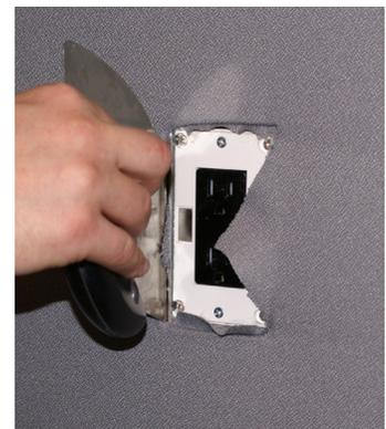
Next, use a putty knife, or similar, to tuck the fabric between the outside of the enclosure box and the MDF.
