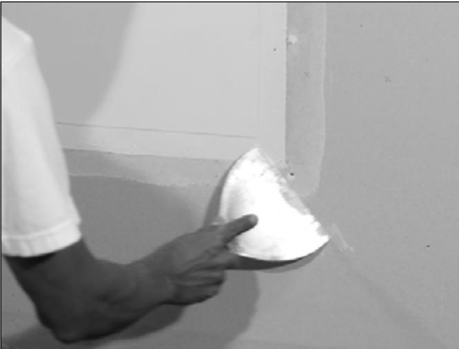
3. Allow hot mud to set slightly before applying mesh tape.
