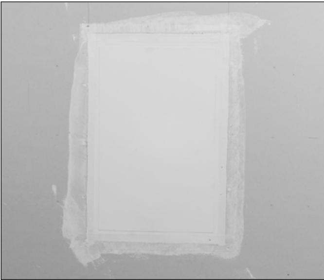
8. Feather all surfaces around the joints and up to the raised portion of the speaker diaphragm.
