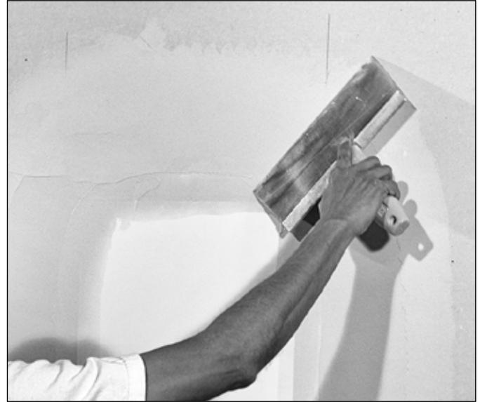
7. Once hot mud has fully cured, cover joints with slow-setting compound.
