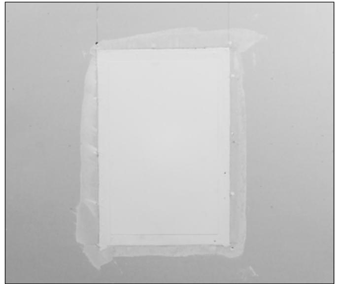
4. Place mesh tape over the drywall seams. Overlap tape slightly.
