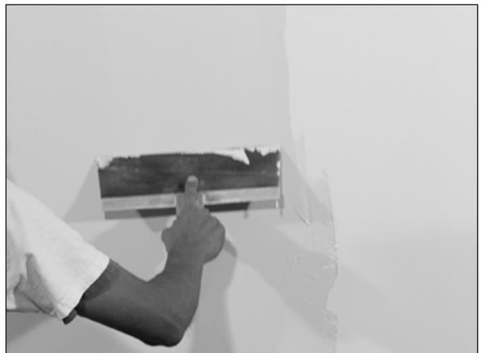
15. After final coat is applied and has dried, use a manual pole sander or block sander on entire wall (do not use a power sander as this could damage the surface of the speaker). Be careful not to sand down into the surface of the speaker. This could damage the paper which makes perfect blending very difficult to achieve. Wall surface should show no signs of a speaker.
