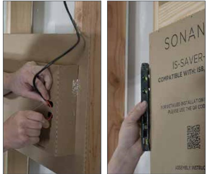
5. Complete drywall installation to the rest of the room including the surface around the speakers. **NOTE: Sonance recommends using the included stainless steel screws around the speaker locations. This is to avoid interfering with the Sonance DISC system depth gauge operation after install. Though this is not required, it will improve the accuracy of finish thickness measurements later on.**
