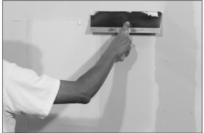
12. Detail the compound to minimize tool marks.
