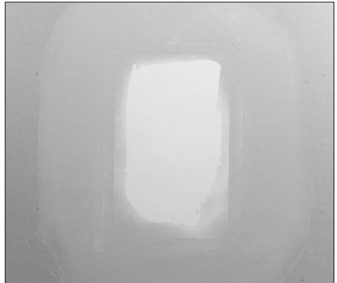
**NOTE: DO NOT use fast-setting drywall compound (“hot mud”) to cover the speaker; it is not flexible enough to provide a durable finish for invisible speakers. Instead we recommend a lightweight all-purpose joint compound to cover joints and feather up to the surface of the speaker. Lightweight, easy-sand topping compound should be used for covering the speaker.**
