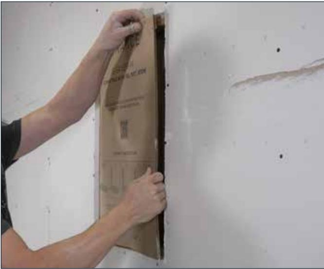
8. **OPTIONAL:** If the zip ring was also used, cut the drywall at the speaker location using a zip tool and the zip ring as a guide. Be sure to cut along the outside edge of the zip ring. It will stay in place permanently.
